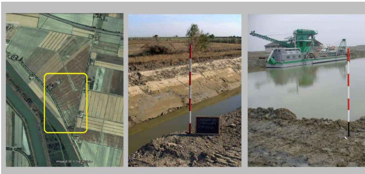
Fig.I.1.5 - Example of workflow sequences in San Giovanni di Ostellato, Cantoniera Cavallara. On the left, a satellite image of the quarry area before the start of the work (image 2016 Digital Globe) with clear soil markers of the main riverbed meander; excavation of an exploratory trench for detailed stratigraphic analysis; positioning of the first dredge in the water.
