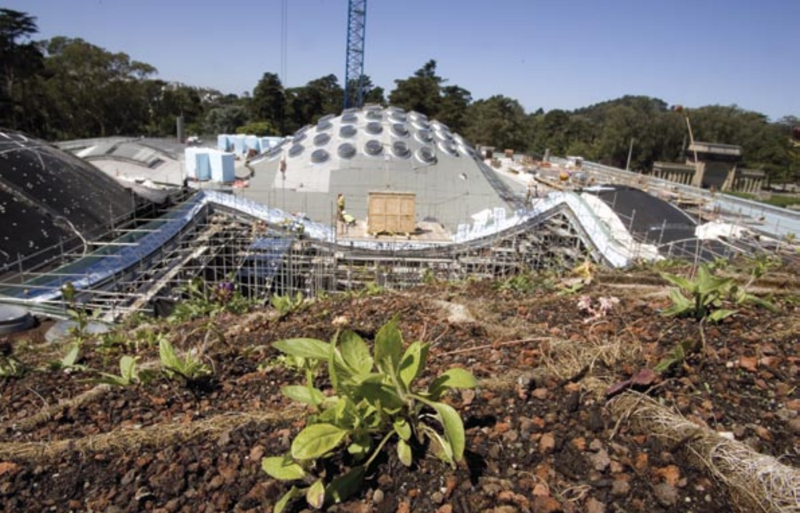
Figura IV.32: Vista del cantiere Fonte: http://greenarchitecturenotes.com/2009/04/a-success-story/
